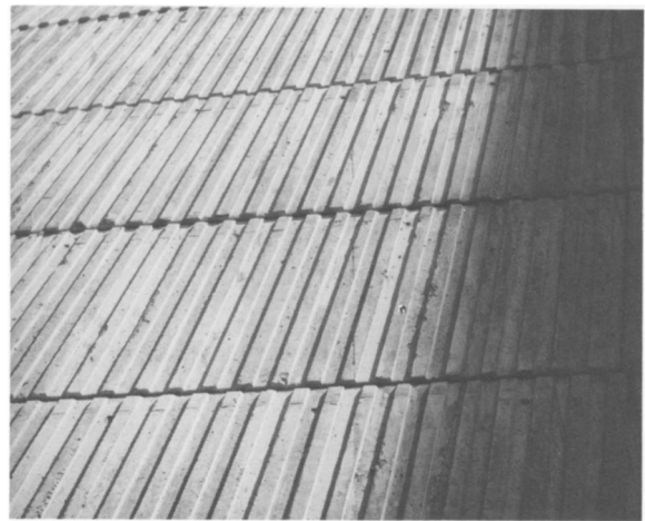
Detail showing texture of hyperbolic paraboloid walls.
