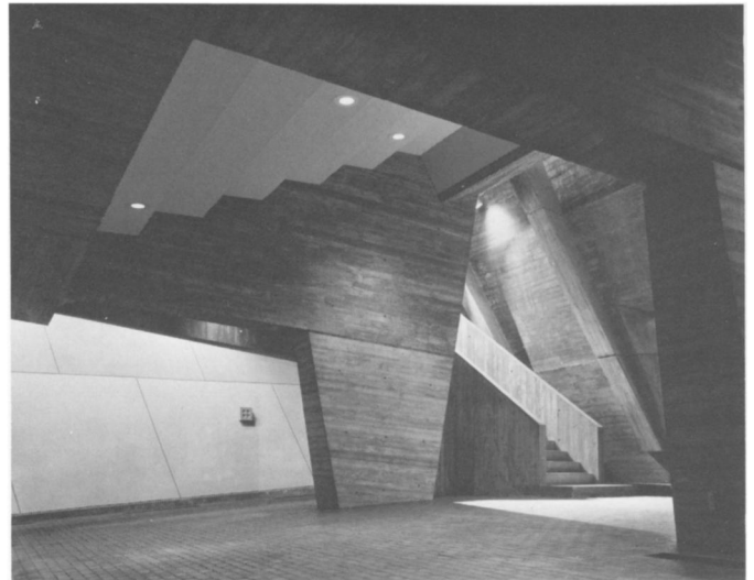
Structural supports of balcony with access stair.
